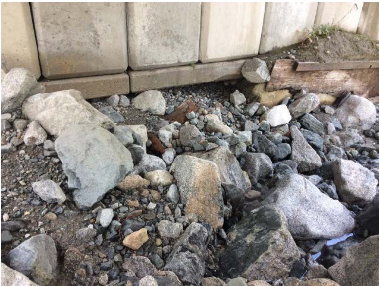
Left Bank Abutment when facing downstream
