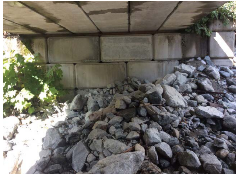
Right Bank Abutment when facing downstream
