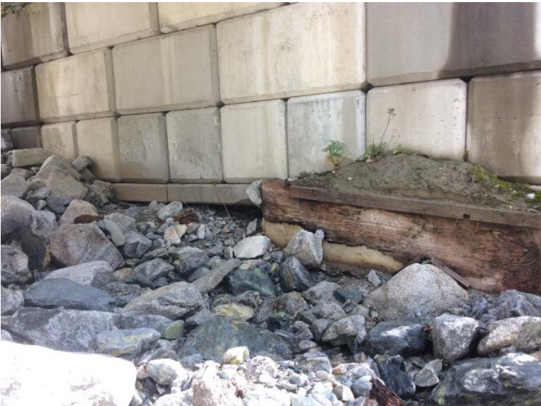
Left Bank Abutment when facing downstream
