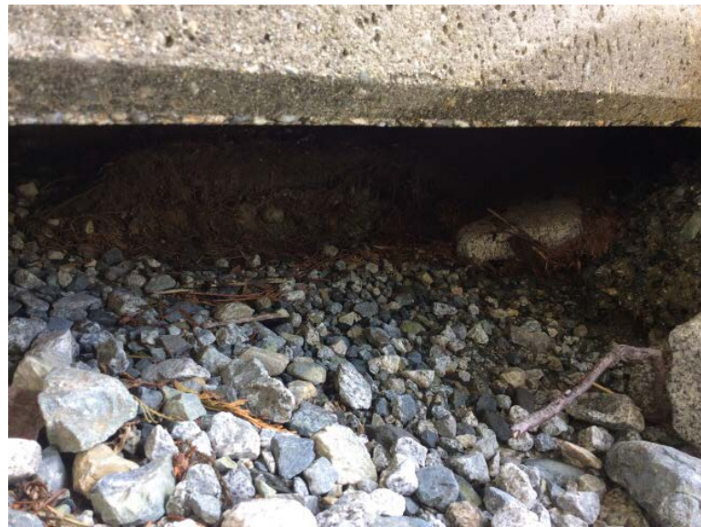
Left Bank Abutment when facing downstream
